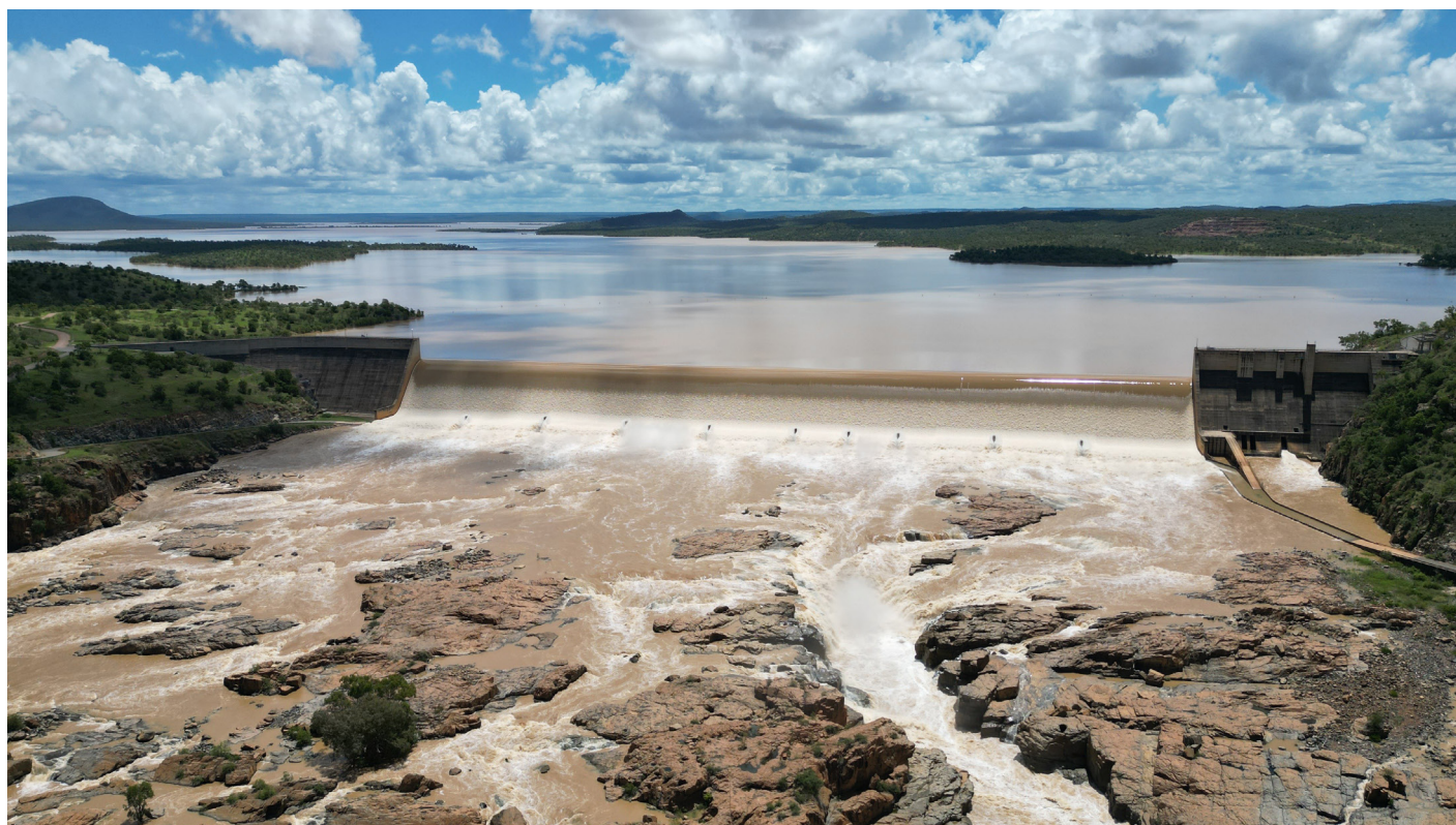
Burdekin Falls Dam spilling
